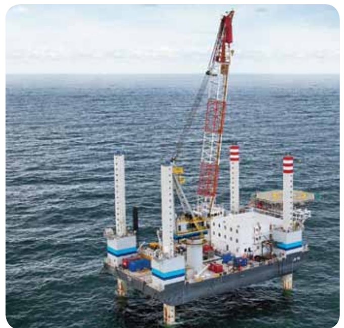
A marine exclusion zone will apply around the jack up barge at all times during construction.
