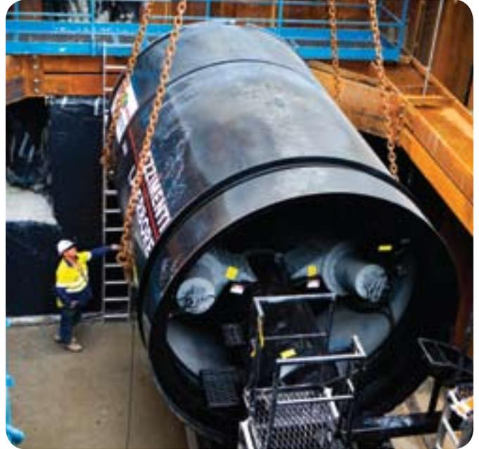
The underground boring machine is lowered into the shaft.
